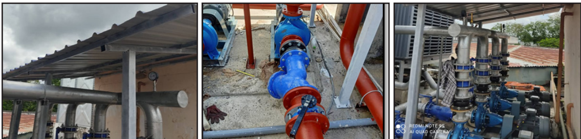
Gambar Kemajuan Penggantian Sistem Water Cooled Package (Fasa 1)
